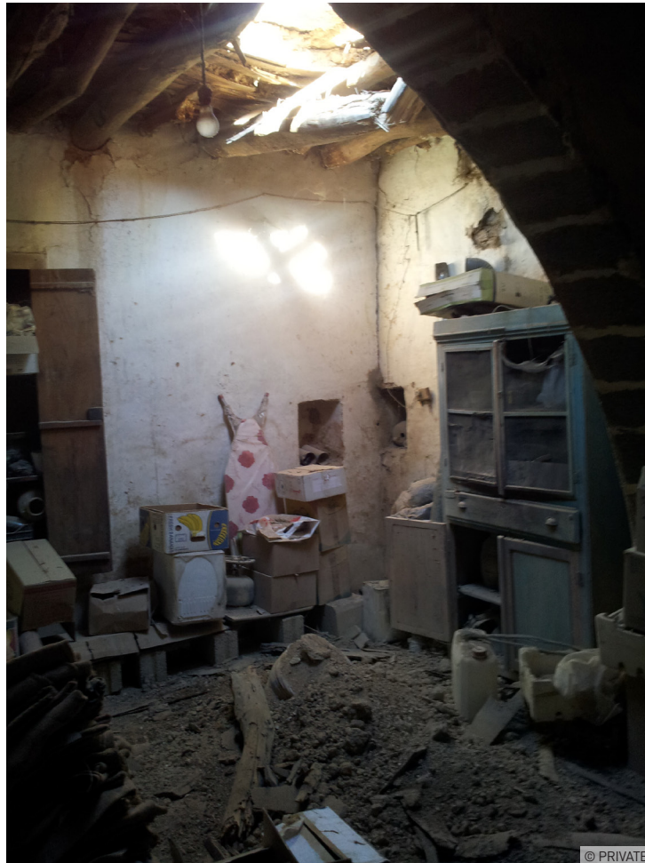
Figure 5: Effects of shelling on a home in Daraya during the August 2012 attack
