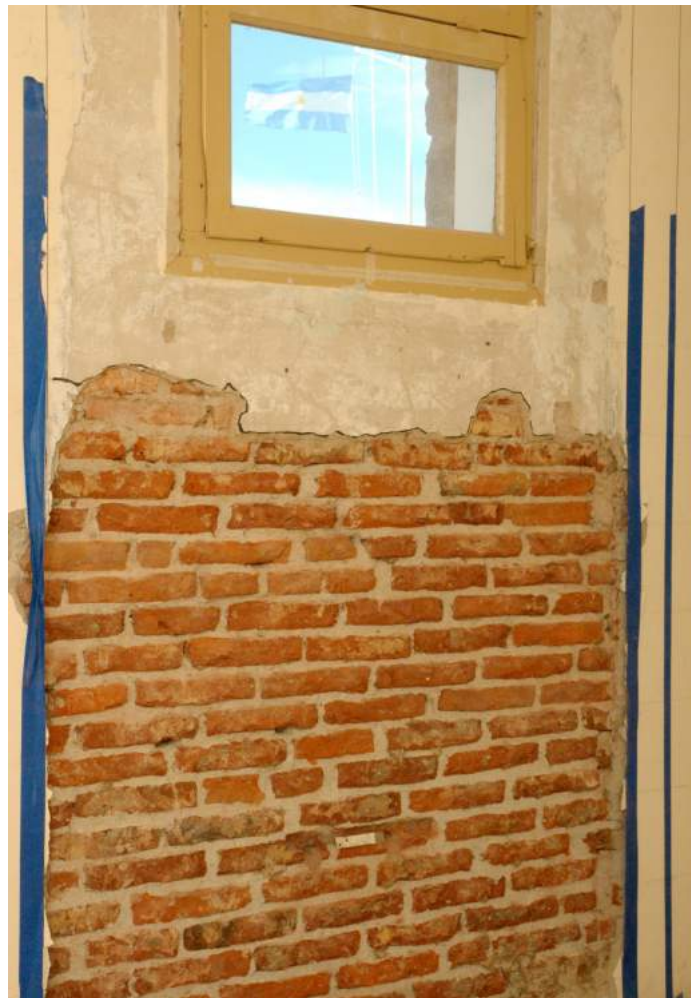
Figure 33 Paint layers found in distinct end wall areas. Beyond the 1.70-m line, the sequence is equal to the upper part of the rest of the main hall.
