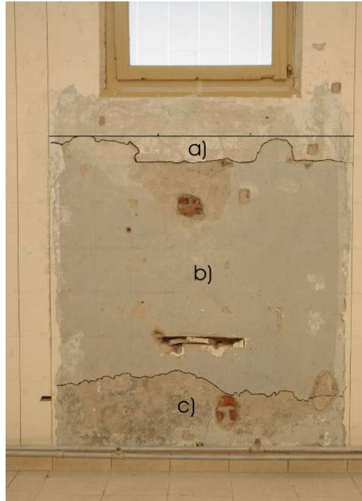
Figure 22 Paint layers found in distinct areas of the far north wall. Beyond the 1.70-m line, the sequence is the same as that on the upper part of the rest of the main hall. Zones with different paint layer sequences in the far north wall: (a)Upper area: between the horizontal line at 1.70 m from the floor and a lower irregular limit marked in black. The wall kept remnants of primer. (b)Intermediate area: between two irregular borders. The wall was painted in light gray. (c)Lower area: from the bottom edge of the intermediate zone to the floor. The wall was painted in dark gray. Above the 1.70 m line the sequence of paint layers also changes.
