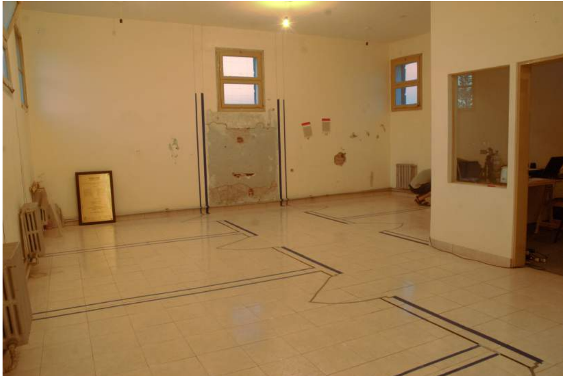
Figure 18 Reconstruction of the walls that took place on-site. This is the step prior to the drafting of the floor plan.
