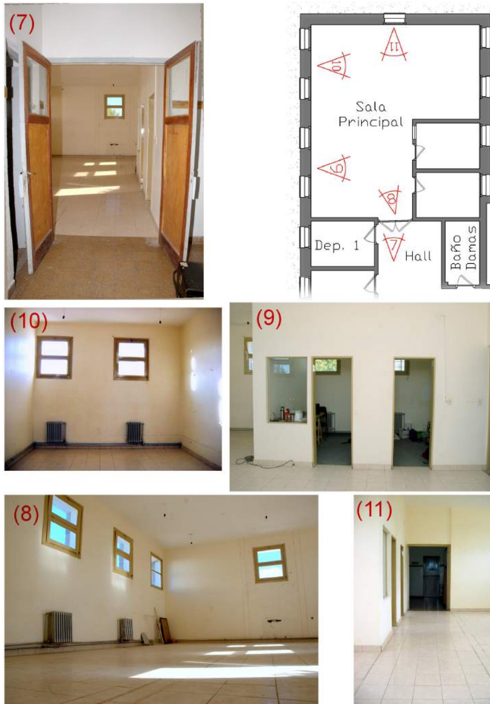
Figure 6 Photos of the main building. West wing.
