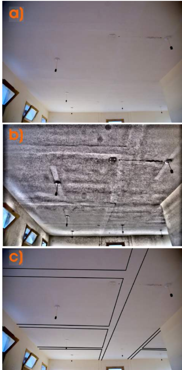
Figure 16 (a)Photo of the ceiling of the main room, facing the northern side. (b) The same picture, with local contrast highlights. The original position of the walls can be seen, as well as lamps hanging from electrical boxes, and marks left by tube fixtures. (c) The original picture, plus the ceiling lines that were observed though contrast imaging in picture (b).
