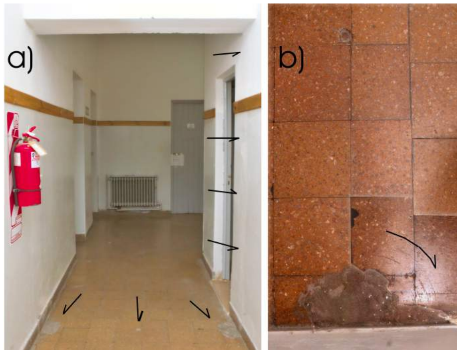
Figure 13 Evidence of the now-removed entrance door in the west wing. (a) View from the entrance hallway that led to the cells. The three marks on the floor can be seen, as well as the irregular wall on the vertical line of the marks. (b) Floor detail on the side of the current ladies' bathroom, showing prints left by a moving door rubbing against the tiles.
