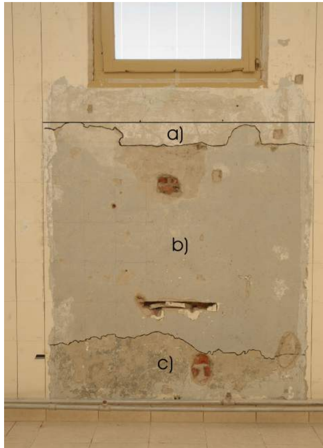
Figure 29 Paint layers found in distinct areas of the far north wall. Beyond the 1.70-m line, the sequence is the same as that on the upper part of the rest of the main hall. Zones with different paint layer sequences in the far north wall: (a)Upper area: between the horizontal line at 1.70 m from the floor and a lower irregular limit marked in black. The wall kept remnants of primer. (b)Intermediate area: between two irregular borders. The wall was painted in light gray. (c)Lower area: from the bottom edge of the intermediate zone to the floor. The wall was painted in dark gray. Above the 1.70 m line the sequence of paint layers also changes.
