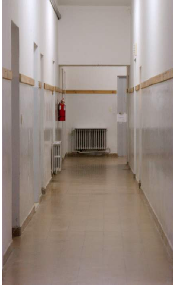
Figure 8 Entrance hallway to the west wing. Photo taken from the entrance hall, in the direction of the main room. The wood trim that conceals the difference between the paints below and above 1.70 meters from the floor is visible.
