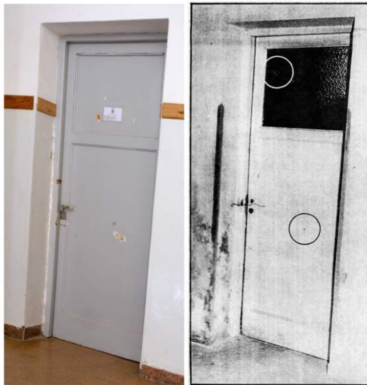
Figure 34 Two pictures of the bathroom door: (left) the current one, and (right) in 1972.
