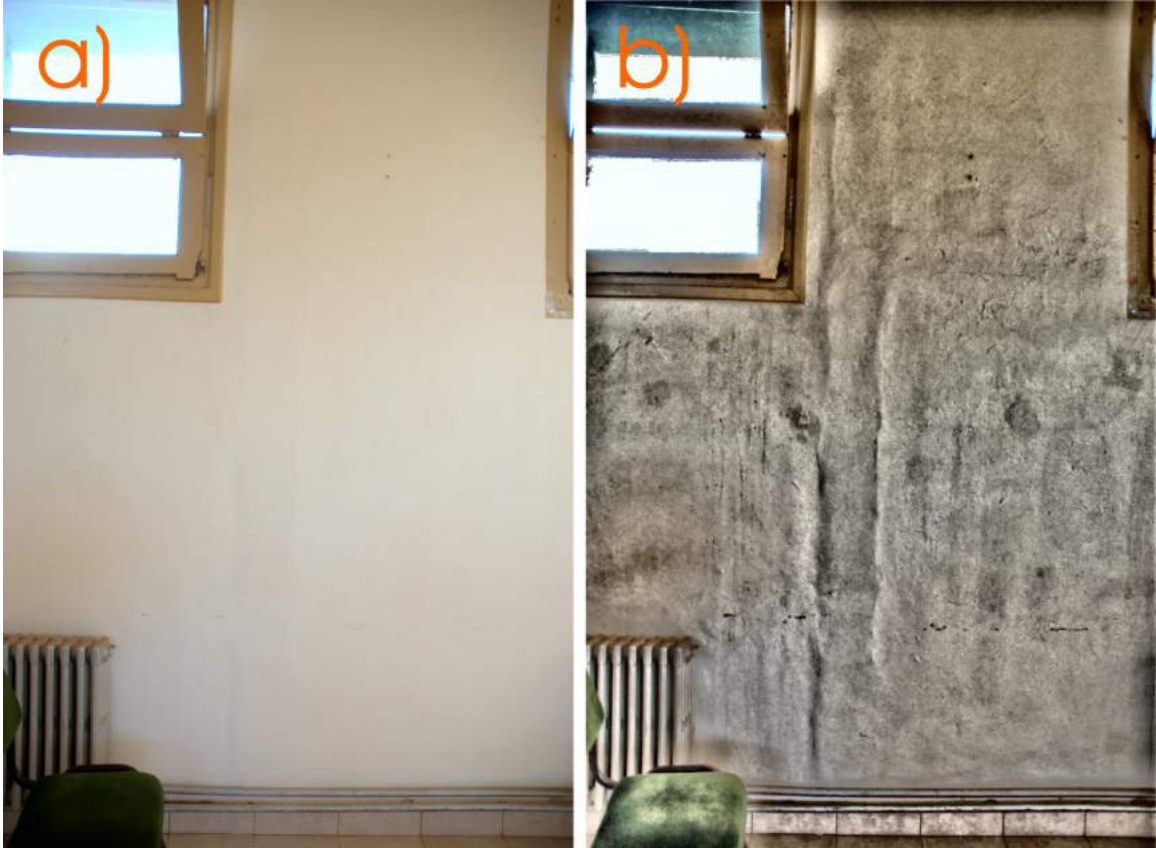
Figure 15 (a) Picture of the west wall in the main room. (b) The same picture after applying a highlight of local contrast. Note how the position of the wall becomes visible, as well as other repairs, imperfections, and small damages that passed unnoticed in the original picture.
